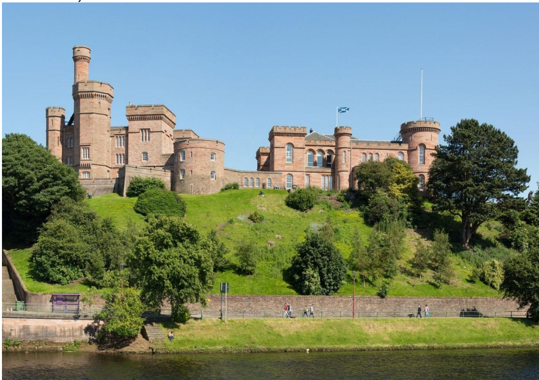
PLATE 2: VIEW FROM WEST, ACROSS THE RIVER NESS: 1840s BLOCK ON THE LEFT; MAIN COURTHOUSE ON THE RIGHT
